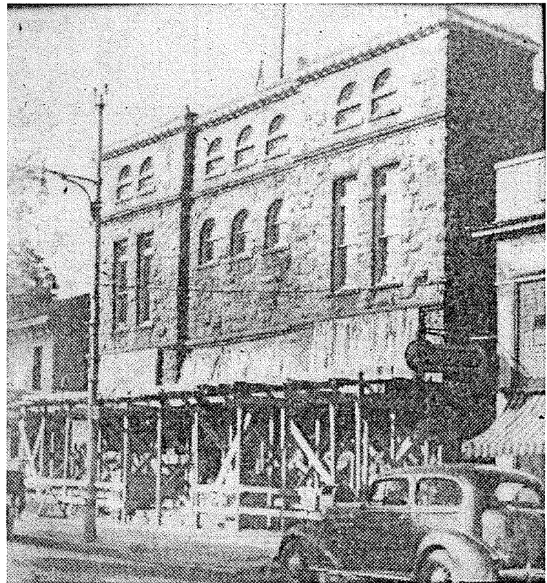
Figure 5. Repair work being done to the front stone work of the Massena Town Hall. The stone work bulged outward on the front bottom third as a result of the earthquake. The picture is from page 14 of the September 18, 1944 Watertown (NY) Daily Times (Tour Stop #10).
