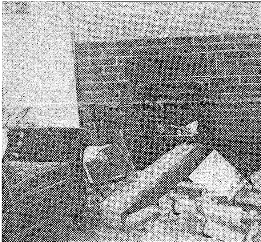
Figure 4. Damaged fireplace in the home of Mr. and Mrs. Charles G. Stubbs, 16 Danforth Place, Massena, New York (Tour Stop #2). The photo is from page 1 of the September 8, 1944 Massena Observer
